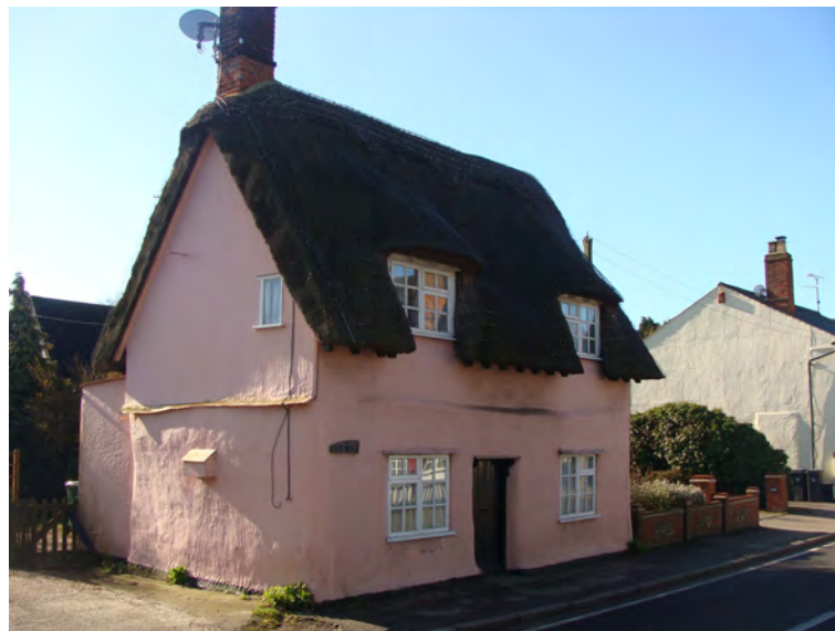
Picture 1.6 Old Neals dating from early 19th century, walls of clay lump to height of about 2.5 m
