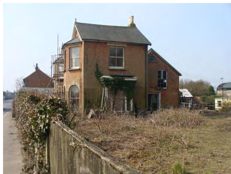
Picture 1.15 Front and north side elevations to Roding Hall. This building should be retained and occupies an important position in the street scene.
